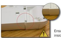
Ensure side rail slots on inside of corner moulding lip.
